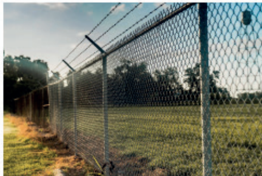
Barbed Wire Fencing
