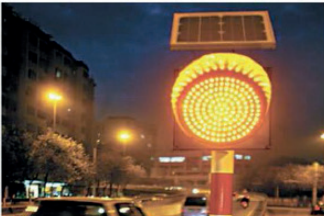
Solar Controlled Warning Lights at Dubai Marina Mall, Pedestrian Bridge
