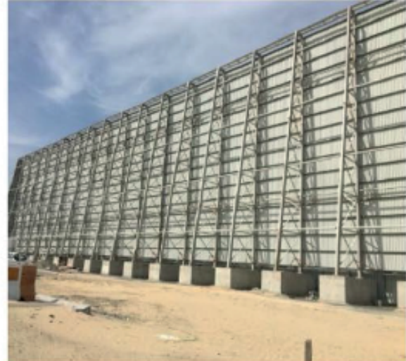
Installation of 105m X 20m Hoarding Board near GEMS School Dubai Hills Estate Site
