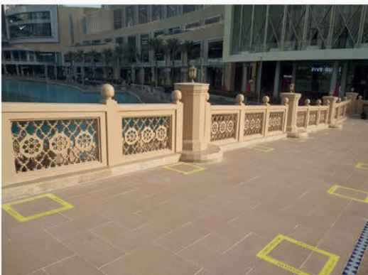
Refurbishment of Souk Al Bahar Bridge at Downtown Dubai Master Community
