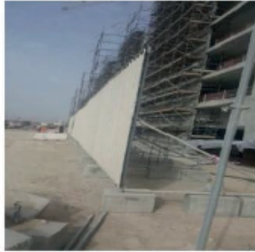
Installation of 4kms Construction Fence at Dubai Hills Estate Construction Site
