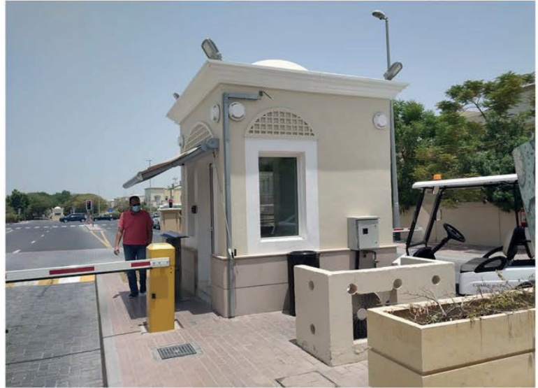
Construction of New Security Gatehouse at Springs Community
