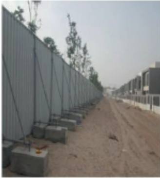
Installation of 4kms Construction Fence at Dubai Hills Estate Construction Site
