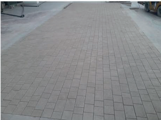
Tegula Tiles Installation at Zone A & C, Dubai Marina Master Community
