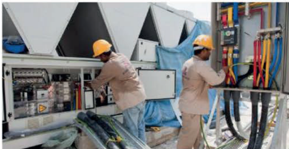
Removal & Supply/Installation of Cables at Arabian Ranches 2
